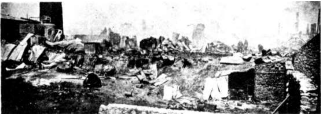
AS SEEN FROM THE EAST SIDE OF BUILDINGS.
