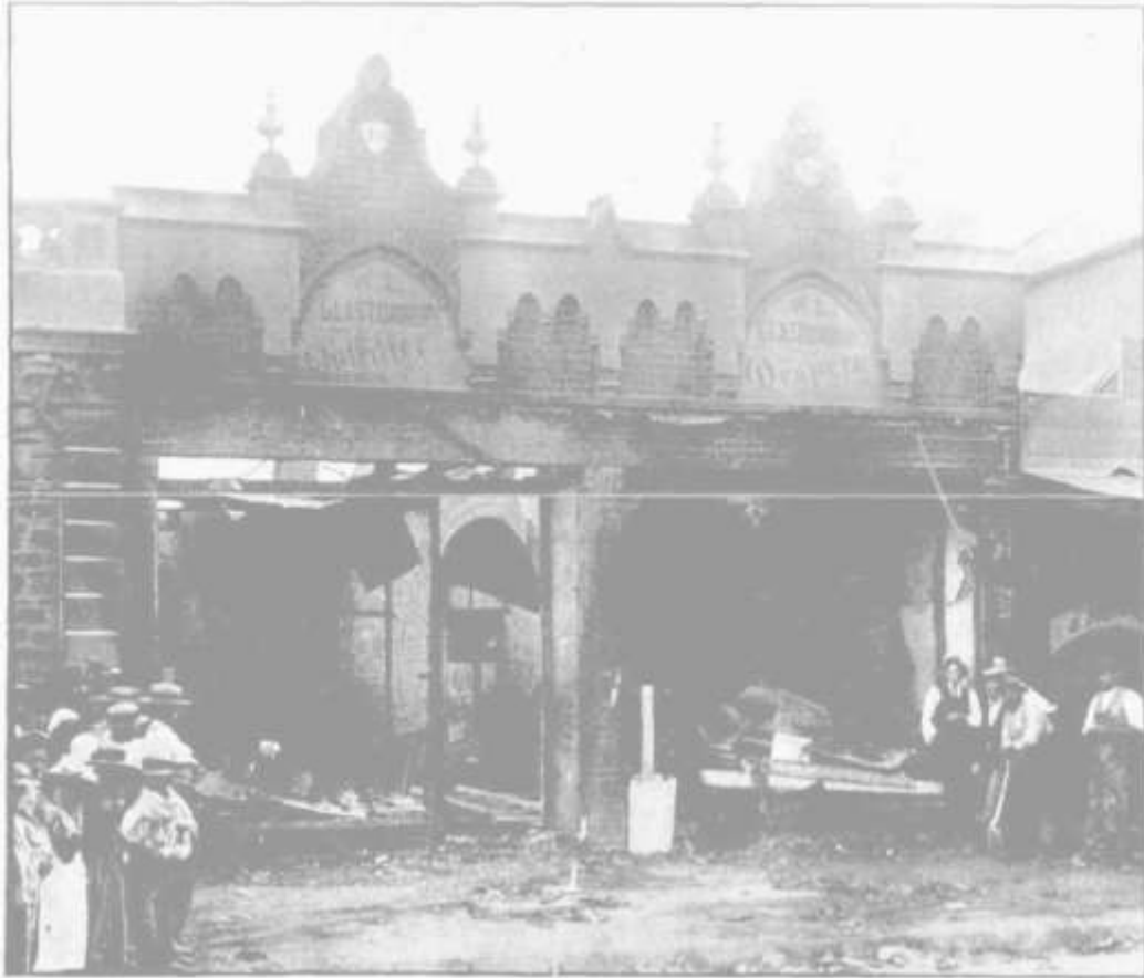
FIRE AT W. L. GLASTONBURY'S SHOP, PORT-ROAD, HINDMARSH. SATURDAY, FEBRUARY 7. THE RUINED BUILDINGS.
